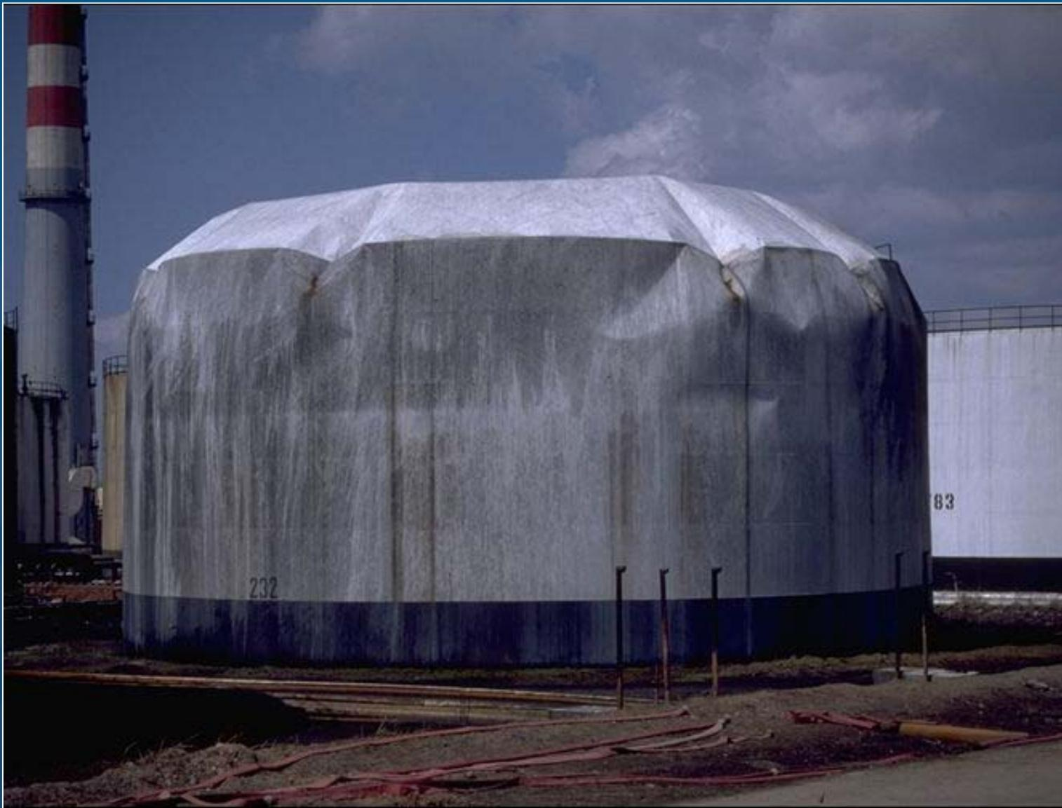
Roof damage in tanks due to liquid slashing
